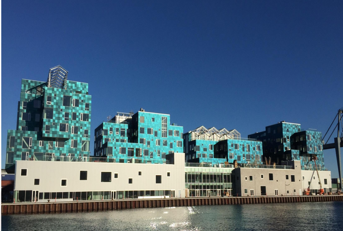
Copenhagen International School 6'600 m 2 | 13'000 Modulen | 720 kW-p
